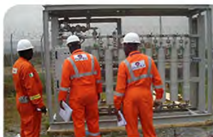
Commissioning of BRT 1 & 2 Nitrogen Generator and Dryer for ExxonMobil
