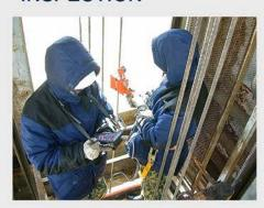
OFFSHORE CRANE ROPE INSPECTION
